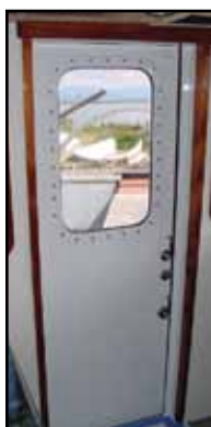
Pilot access, Interior
